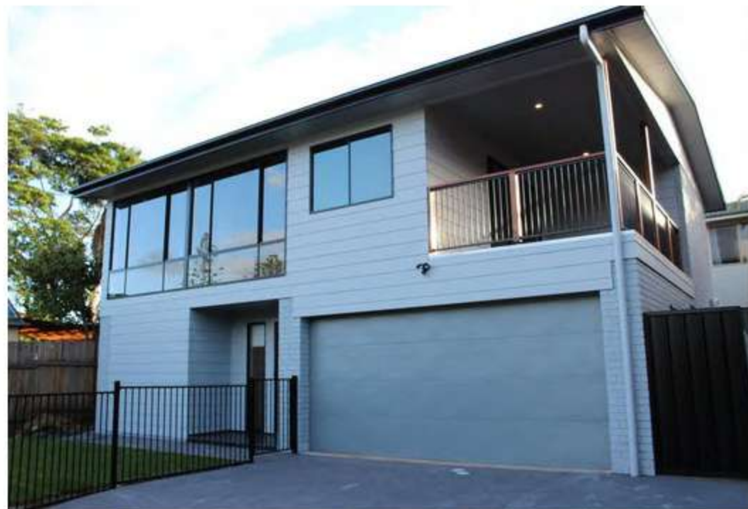
2 Storey Renovation - Port Macquarie NSW
